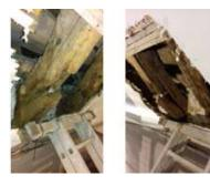
We can replace the rotten rafters with like-for-like timber – hopefully, by the time you get this month's Parish News, the right specialist will be doing the necessary work on the rafters and beams.
